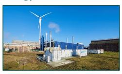
electric vehicle battery packs. Installed at an industrial site, the battery system provides a frequency response service to the local grid operator to help it balance electricity supply and demand for network stability. This is the first time 'second-life' batteries have been used at an industrial scale in this way in the country of Belgium.
